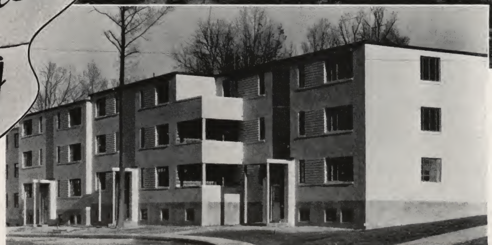
Top —“K” Street Apartments, Washington, D. C., one of four low rent, large scale housing projects built at the national capital by the Alley Dwelling Authority and Public Works Administration. Concrete masonry walls finished with portland cement paint and furred and plastered on the inside. Homer J. Smith, architect. Walter B. Avery, builder.
